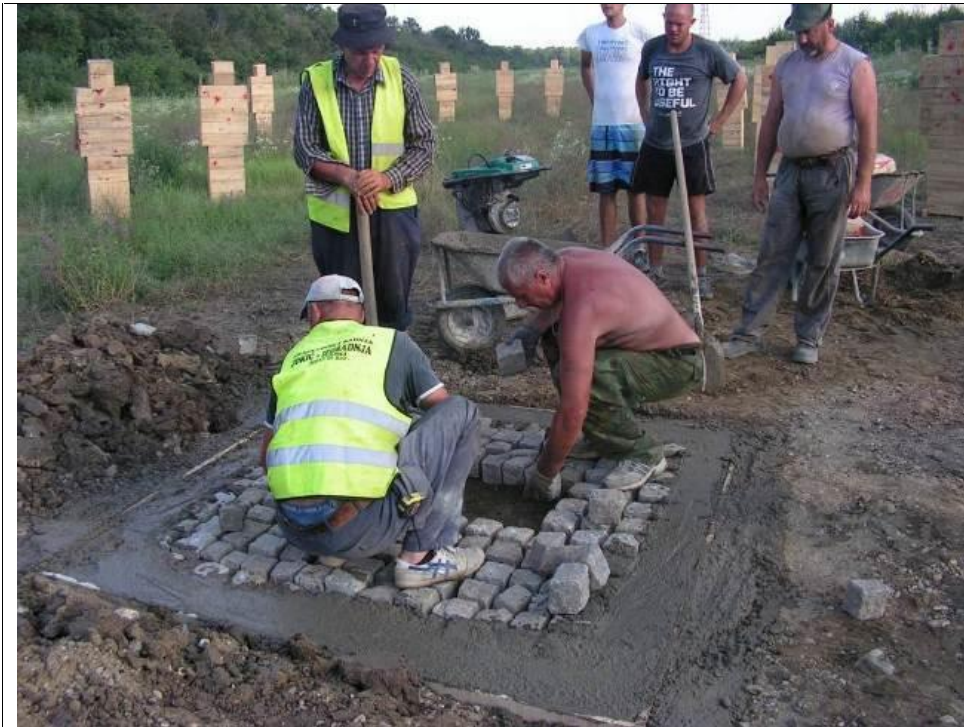
Figure 54 – The making of surface for the activation of explosive
